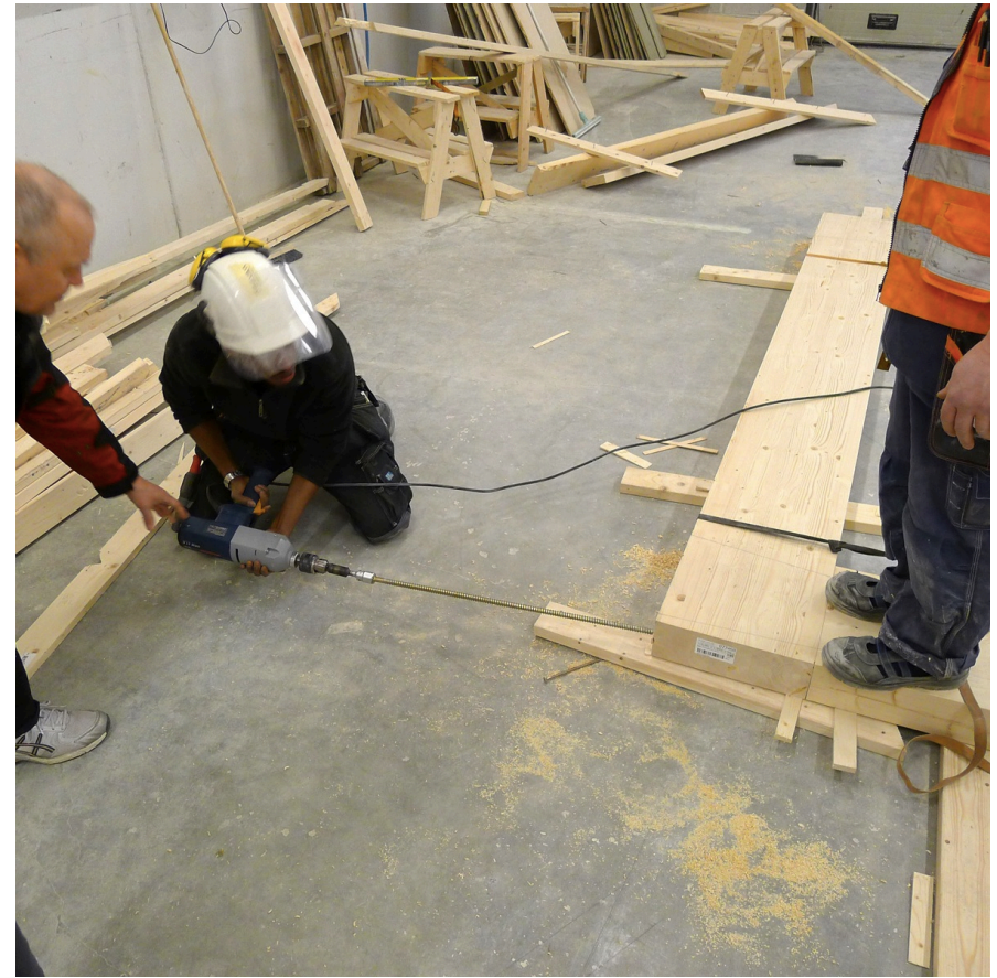
Long screws in corner of glulam frame
